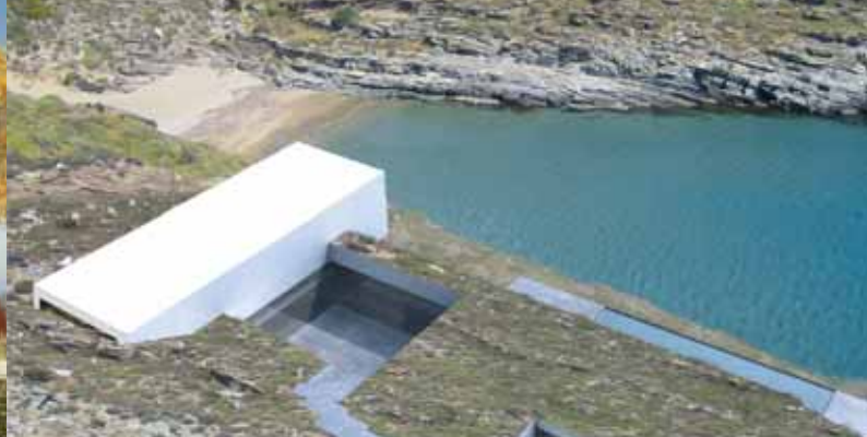
'Xiroliitha' Summer House A hidden, courtyard house with a single stone façade topped by a white block. Inspired by the stone walls of the Greek Islands.
