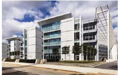
**Network Rail, Milton Keynes** The Quadrant:MK is Network Rail's national centre and accommodates some 3,000 staff in four buildings linked by a central atrium. It is highly energy efficient and uses natural ventilation combined with the building orientation and solar shading to minimize the energy used for heating and cooling.
