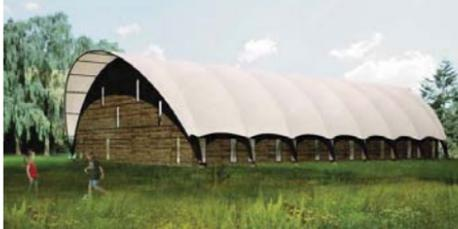
**Light arena construction, Ringe** Multi sports arena of round steel beams covered by translucent membrane. Area 800m<sup>2</sup>, built 2012.
