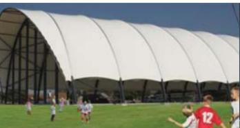
**Unheated multi arena** Curved steel rafters and a light membrane allow daylight through. Large gates facilitate a variety of applications.
