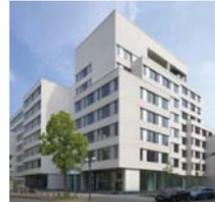
Revitalisation project: Office building Feldbergstrasse 35, Frankfurt am Main An award-winning project with a total of 8,000m<sup>2</sup> gross floor area. To maximise the usability and sharpen the character of the building, newly developed air conditioning units with a digital slit pattern were introduced into the façade design. Completion 2009.
