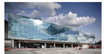
**Infrastructure: Dublin Airport Terminal One Extension** Phased design development, management and construction of an ADR designed two-storey extension elevated on columns.
