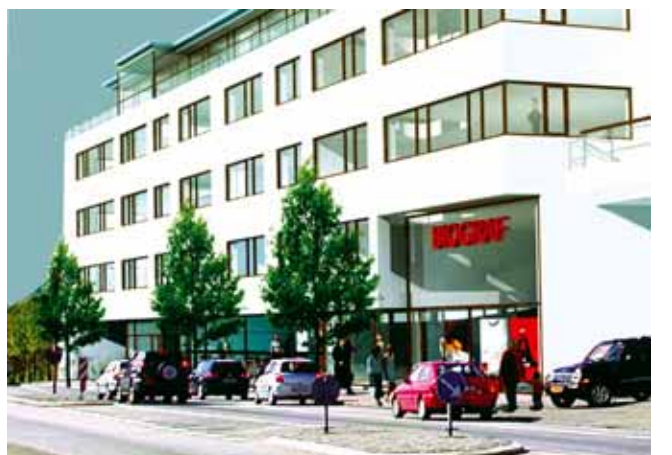
Statoil, Copenhagen Apartments, a cinema and multi-storey car parking for Elsoe-Ejendomme. 10,000m 2 gross for completion in 2008.
