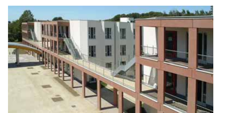
3rd Generation Accommodation, Brussels A hospitality establishment with 217 beds including 37 apartments for elderly, but able people.
