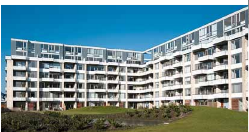
Tegholms Have, South Harbour, Copenhagen 142 full-ownership apartments for MT Højgaard. 12,600m 2 gross completed in 2006.
