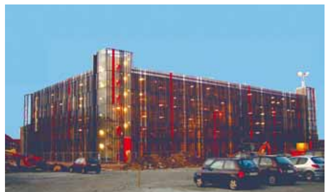
Multi-storey car park, South Harbour, Copenhagen Completion in 2007 for Zeta Park. 15,000m 2 gross with space for 667 cars.
