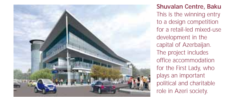
Shuvalan Centre, Baku This is the winning entry to a design competition for a retail-led mixed-use development in the capital of Azerbaijan. The project includes office accommodation for the First Lady, who plays an important political and charitable role in Azeri society.
